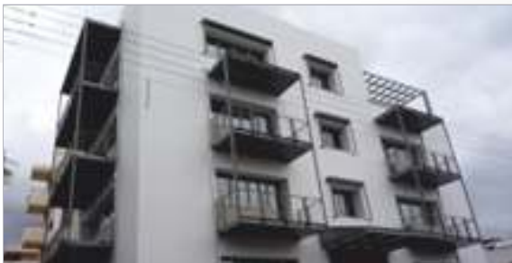
Office building, Holargos - 1,500 m 2 .
