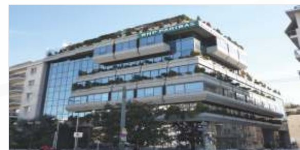
Office building, Vas. Sofias 94 - 7,800 m 2
