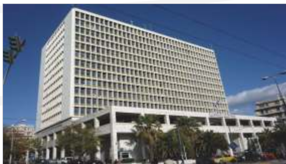
General Attica Police Department, Athens - 30,000 m 2
