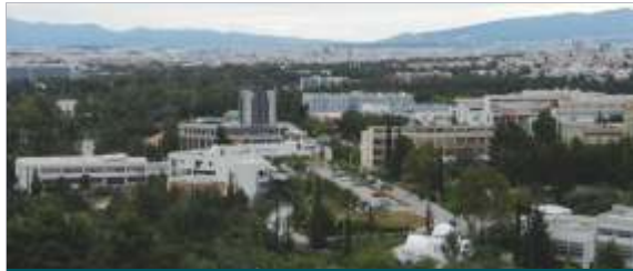
NTUA, Energy monitoring of the 22 buildings on campus, 50 monitors
