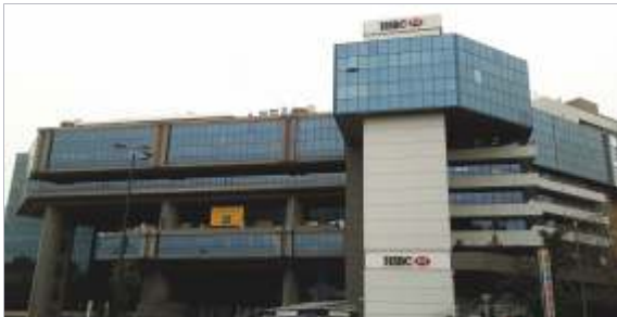
Office building, Mesogeion Str. 109 - 111 - 1,900 m 2
