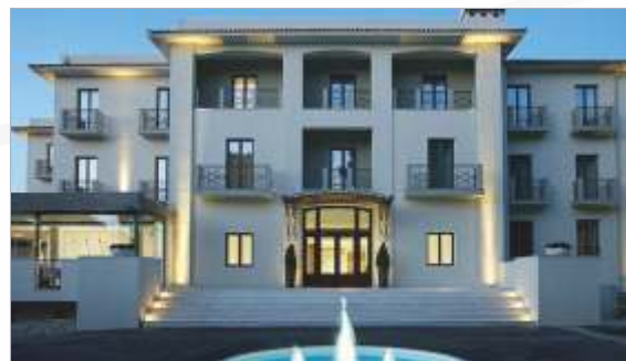
Domotel - Educational Centre and Hotel 16,000 m 2 , 1,400 control points
